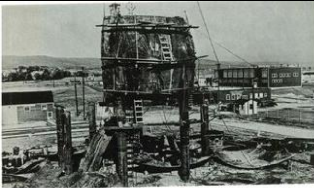
A test sphere that enabled the investigation of effect of agent was constructed during the early 50's and greatly improved existing sampling and dissemination techniques.
